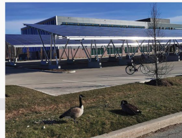
Solar panels covering the evolv1 parking lot
